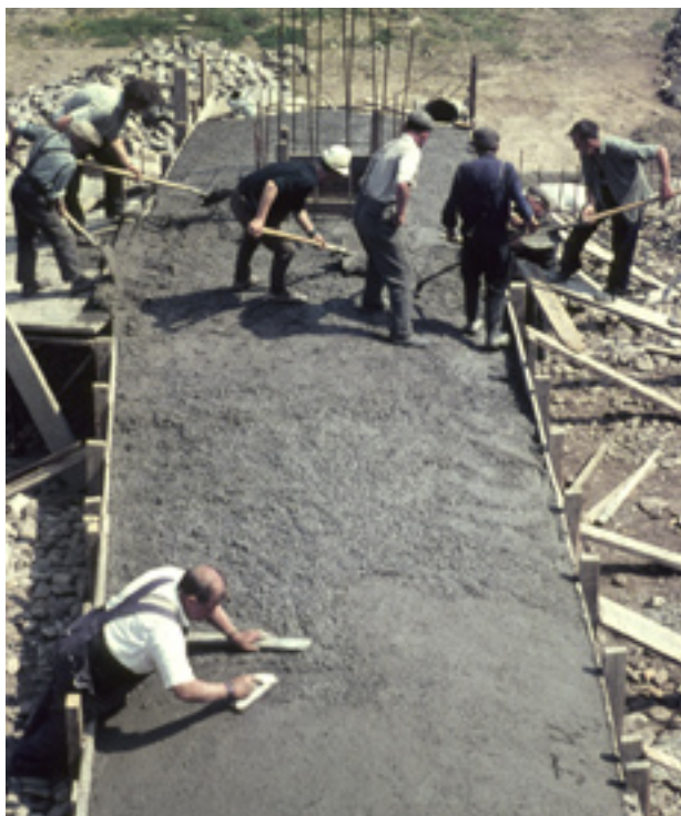
Fig. 3.26: Spreading the concrete capping over the passage at Newgrange [O'Kelly archive, DoEHLG]
