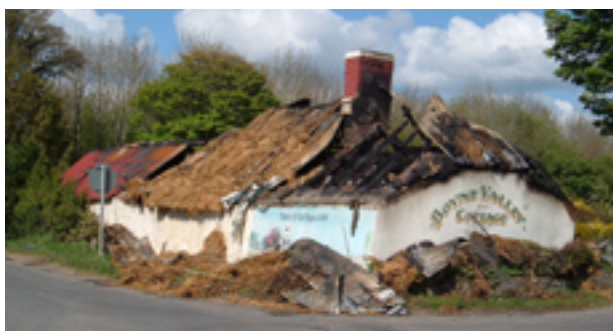
Fig. 3.25: Boyne Valley Cottage, Donore, before and after a fire in May 2008 [Jill Chadwick]
