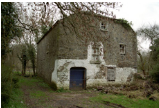
Fig. 2.41: The vernacular mill at Rossnaree occupies the site of an earlier mill run by the Cistercians at Mellifont [Con Brogan]
