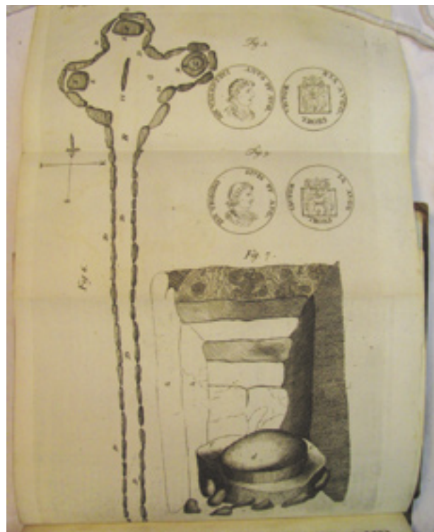
Fig. 1.12: Thomas Molyneux's drawings of Newgrange, published in 1726. His original captions read as follows: Fig. 6 — 'A is the entrance, from A to B the long narrow gallery or passage, eighty feet in length, leading to the cave C. DDDDD the great flag-stones that make the sides or wall both of the cave and entrance. EEE the three cells or apartments let into the sides of the cave, for the convenient reception of the three altars or shallow cisterns, FFF G a second altar, raised upon the lower altar in the right hand cell. H a pyramid stone now fallen, but formerly set up erect in the middle of the cave'; Fig. 7 — 'shews more particularly the manner and contrivance of the altar in the right hand cell, consecrated to the deity of Thor, expressing all the rudeness of its wor'; Figs. 8 and 9 — 'shews Valentinian's coin with its reverse... [and] that of Theodosius, both taken from the coins themselves, but larger than the originals, that the inscriptions might be better express' [Image reproduced courtesy of Special Collections, UC'D]
