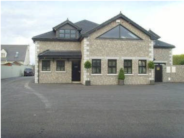
Figure 1 – Building where heat pump is installed
