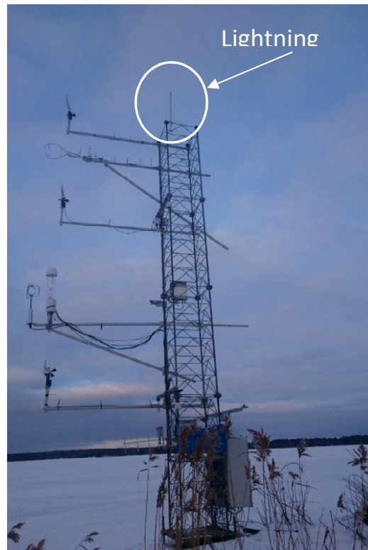
Figure 3. Lightning Rod protecting Gas flux tower on Malma Island, Lake Erken.
