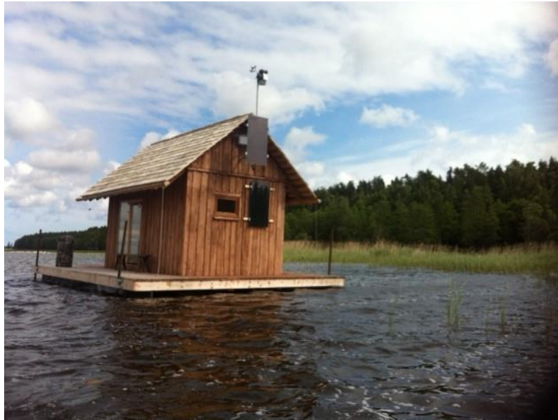
Figure 5. Floating platform as an automated monitoring station.
