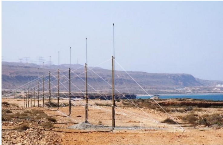
Figure 2.6– Typical land based radar wave measuring system [185]
