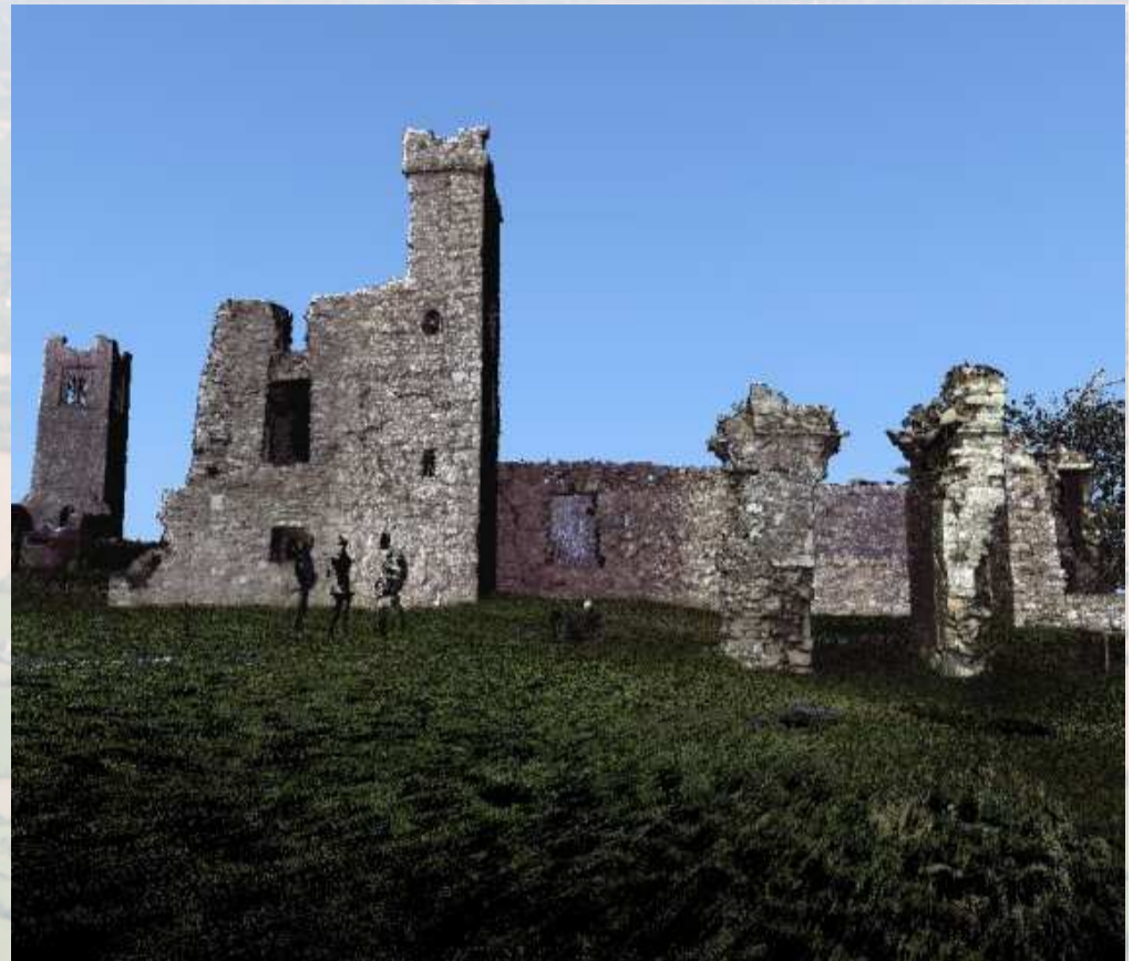
Terrestrial laser scanning; a colour compilation of the scan of the College from the east showing the gatehouse, College wall and the nearby St Patrick's church tower. (The Discovery Programme)
